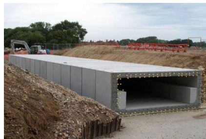
Parramatta Council Stormwater Upgrade
