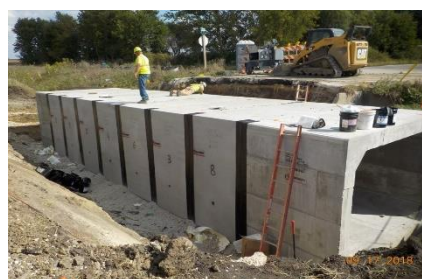
Canterbury Bankstown Council Stormwater work
