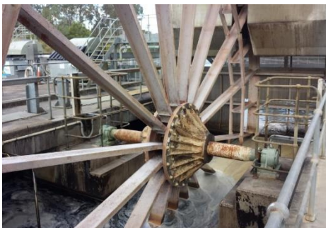
36 Ton Drum Screen Support at SUEZ
