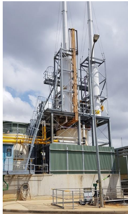
Stability Check of Stack 2 at water Treatment Plant SUEZ
